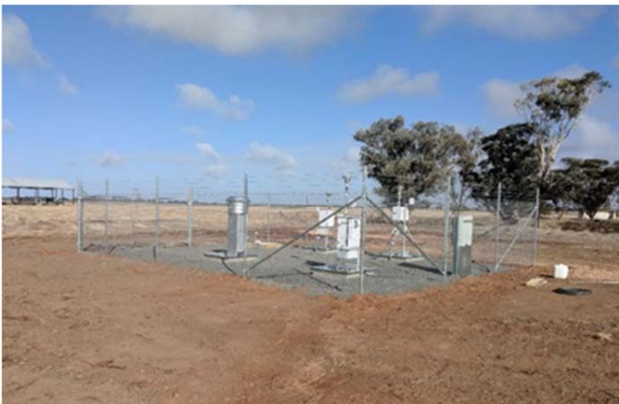
Figure 1: air quality monitoring station
