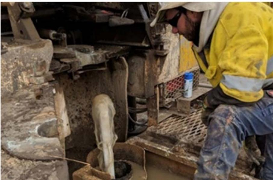
Figure 1: Groundwater monitoring bore installation at Avonbank Project site
