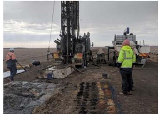
Figure 3: Groundwater monitoring bore installation
