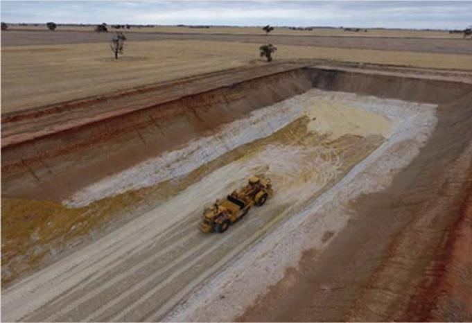
Figure 3: Test pit after stage 1 – overburden capping
