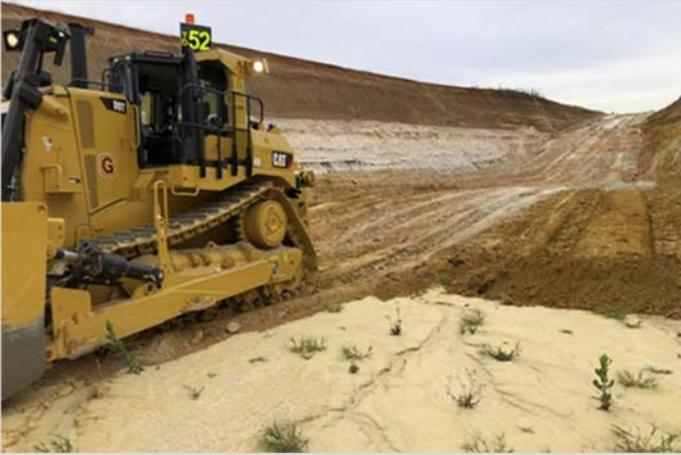
Figure 2: Test pit – tailings being capped by overburden
