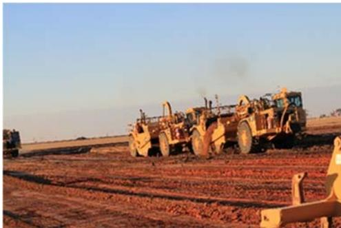
Figure 3: removing topsoil
