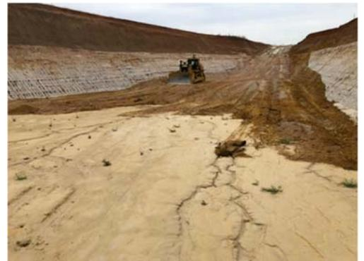
Figure 5: Avonbank overburden being dozer-pushed over the dry tailings
