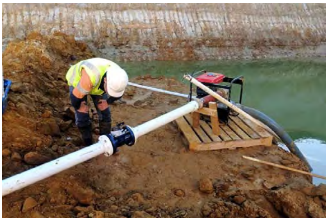
Figure 3: Monitoring ground water flows at the Avonbank Project Test Pit.
