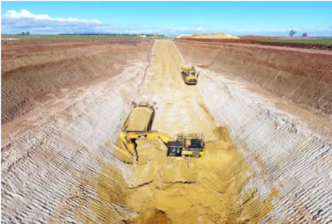
Figure 4: Avonbank Project test pit.
