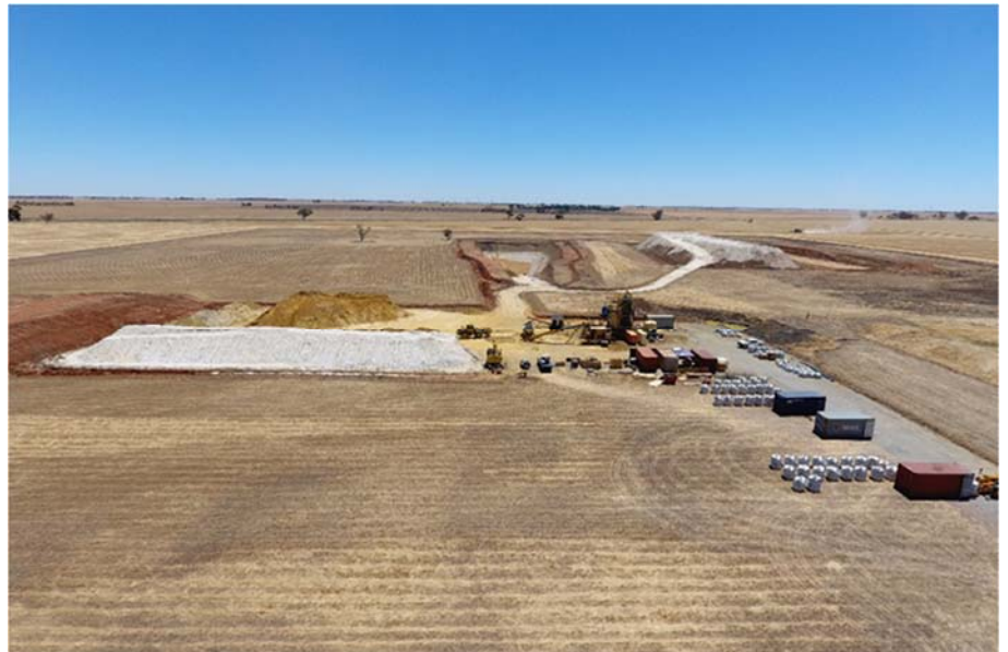
Above: Avonbank Test Pit and Pilot Plant - 2019
