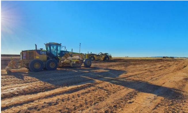
Figure 2: Grading and ripping of sub soil
